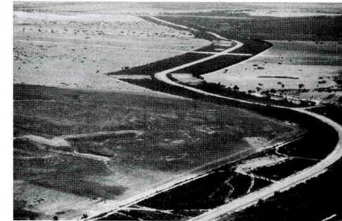
Road corridor, Western Australia, Photo courtesy of B.M.J. (Penny) Hussey.
